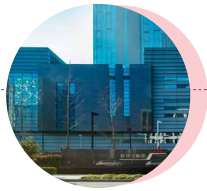
Hangzhou Operation Headquarter/R&D Center
